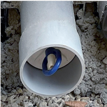
Picture to the left is an example of using the Blank Duct Plug, Inside Fit with Loop Nut.
